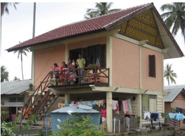
Earthquake- and flood-resistant reconstruction of buildings by the GRC in Indonesia after the tsunami in 2004 Photo: GRC 2008
