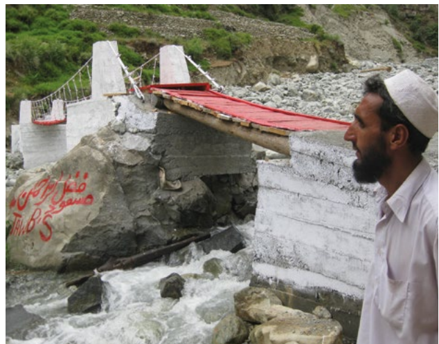
Robust bridges in north-west Pakistan will provide access to villages even during flash floods.
