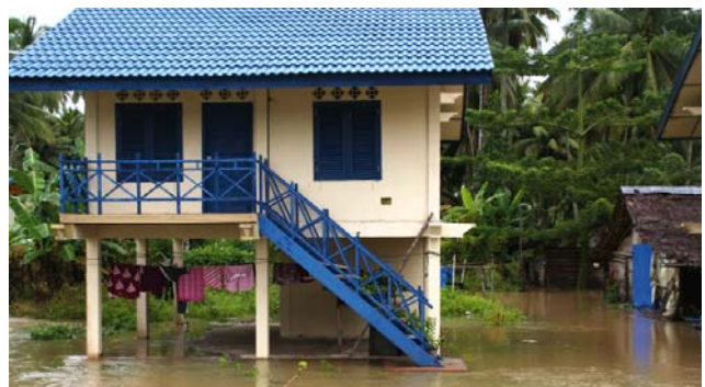
Reconstruction: earthquake resistant and flood proof houses built within a GRC project in Indonesia after the 2004 tsunami.
